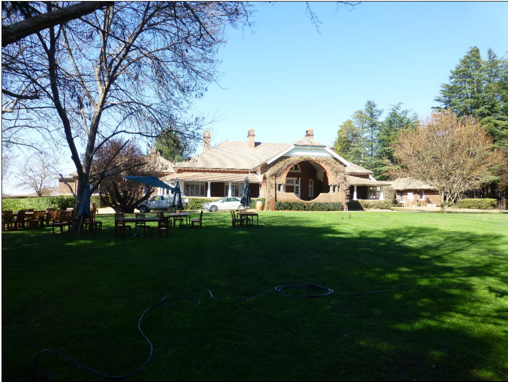
Plate 2: the west-facing face of Palmerston house
